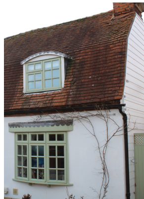
Figure 28 Example of a gambrel roof with dormer window
