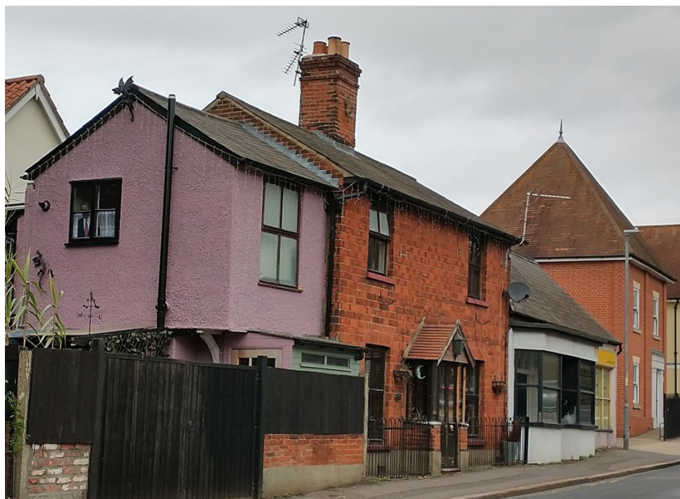
Figure 24 Number 395 Old Road in red brick laid in Rat Trap bond, with numbers 399 and 397 to the north
