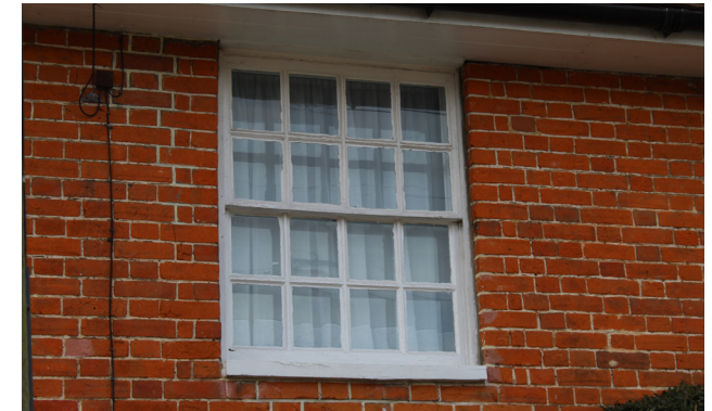
Figure 30 Example of a timber sash window
