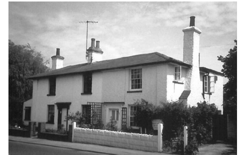
Figure 17 404 and 406 Old Road in 1985 (Essex County Council)
