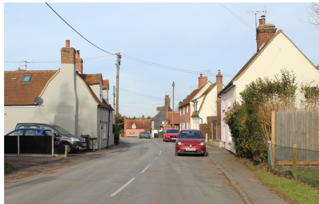
Figure 27 Chimneys and a variety of roof forms add visual interest to the street scene
